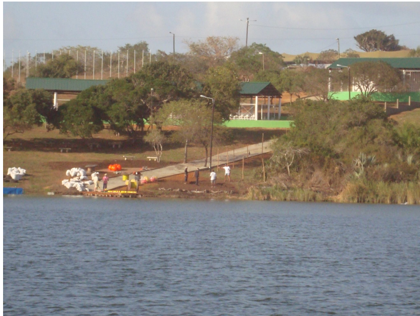
All Africa Games –Venue and Infrastructure Overview
